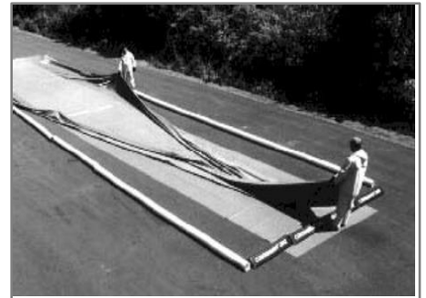
A portable containment pad can be constructed to collect wastewater from power washing. *Photo courtesy of GMC Delco Cleaning Systems.
