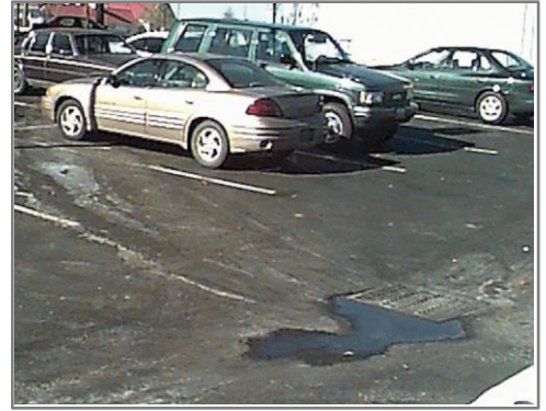
Drains in parking lots usually lead to storm sewers. You CANNOT discharge your power washing wastewater into a storm sewer.
