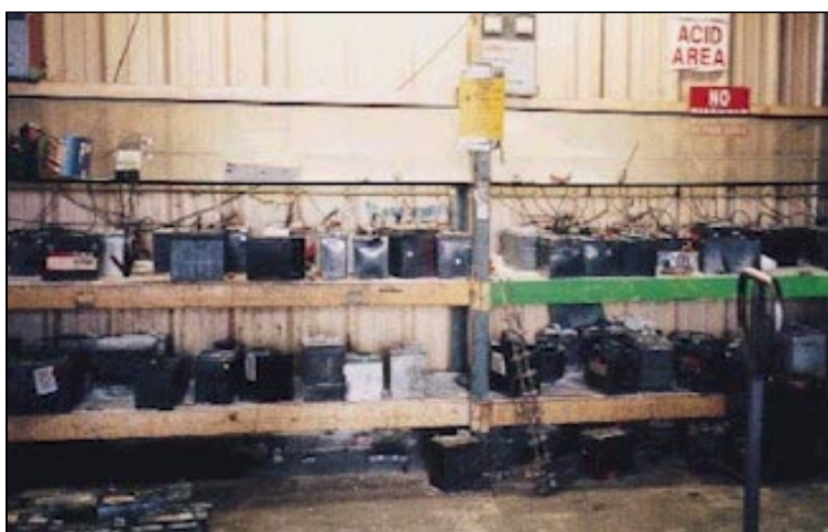
This company has an indoor battery storage area which is well ventilated. An impervious floor helps contain spills and leaks.
