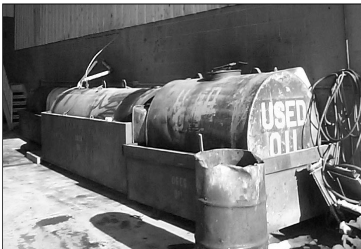
Secondary containment around oil tanks and containers helps to prevent leaks and spills and can help you avoid a costly cleanup.
